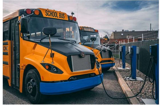
Electric school busses charging 84
