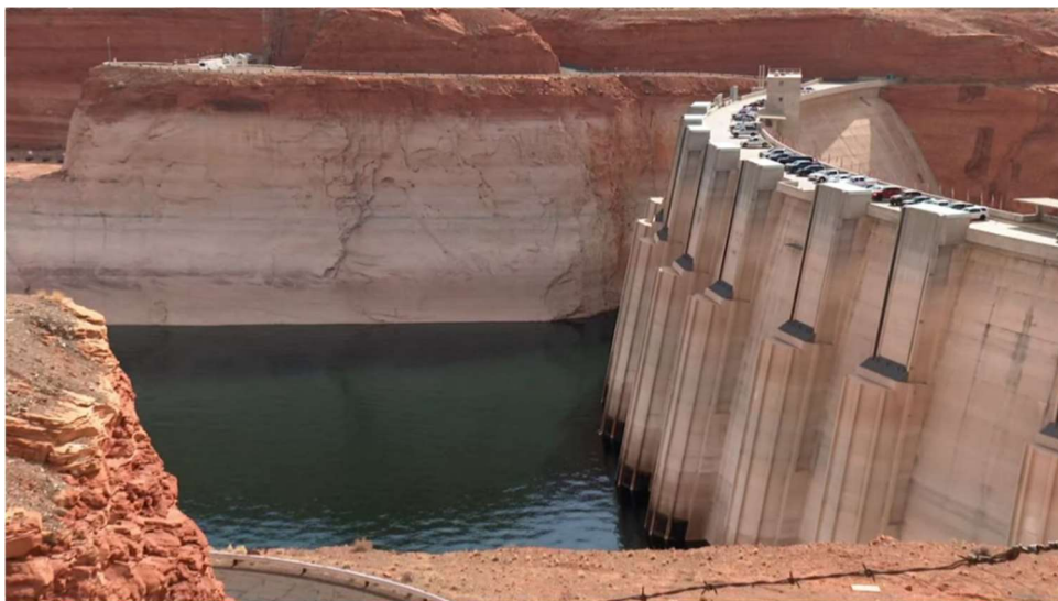
Figure 9- Lake Powell and Glen Canyon dam, April 2022. The white stone indicates where the water levels used to be. Drought and water over-use has caused water levels to drop by over 100 feet over the last 3 years. Power generating capacity has dropped by over 15%. Lose another 32 feet of water depth and electricity cannot be produced from this crucial dam. 16 Regionally, Washington and Idaho have experienced a 10 – 15% reduction in flows through our hydropower dams. Our region is threatened as well.
