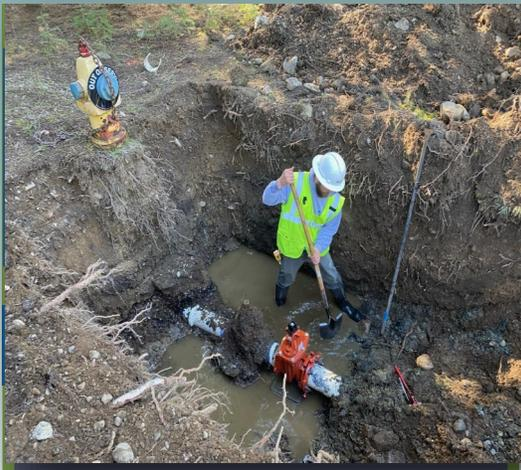
Pictured above is Keenan Olenlager working on a valve replacement for a fire hydrant at Twin Lakes.
