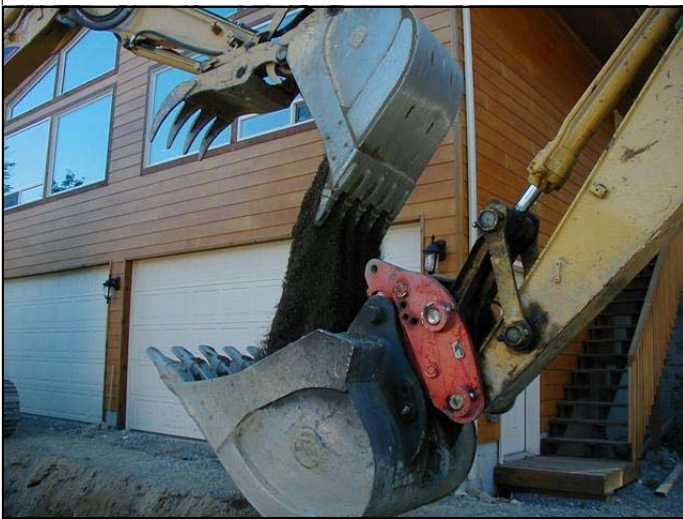
East Tobler Road— Construction Through Narrow Corridor
