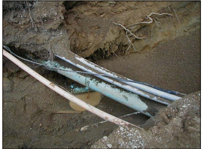
Lower Hayden Lake Road, Existing Utilities
