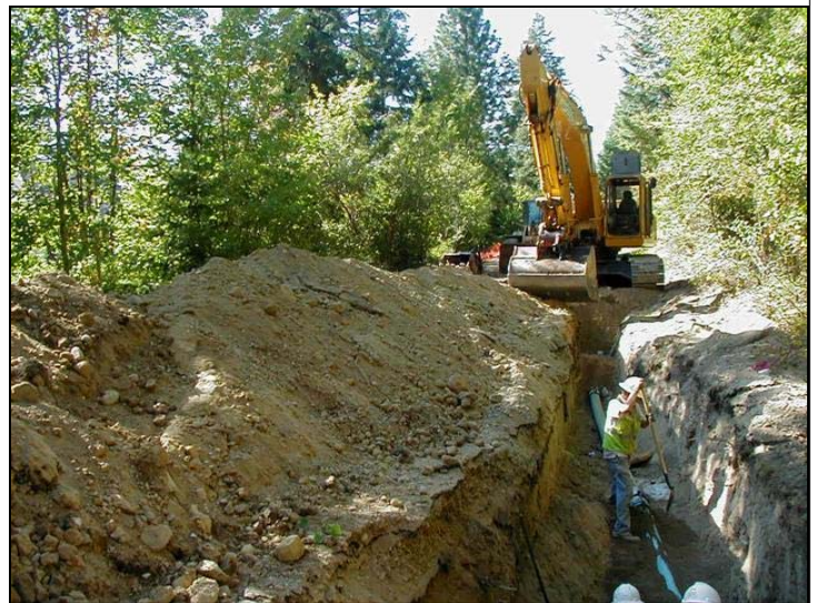
Half Mile to Clarkview, Step Slope Installation
