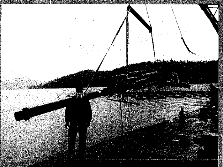
In the picture on the left, Dan Messier, Waste Water Supervisor and on the right, PJ Luckler, O&M Operator, watch from the deck of the barge as they crane lift the intake structure from the lake to repair.
